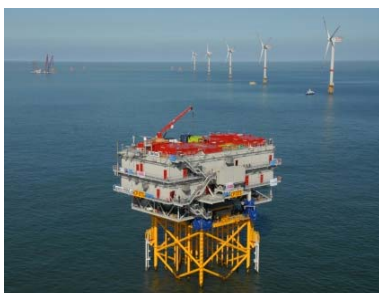
Thornton Bank - installed
