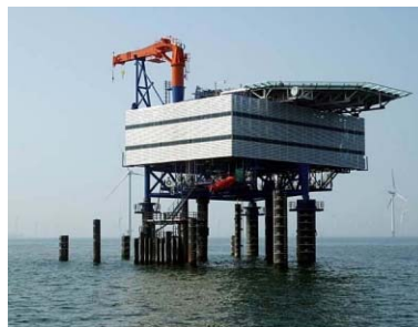
Horns Rev A - installed
