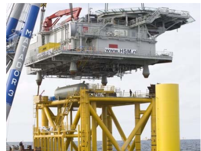
Horns Rev B - installation of top side
