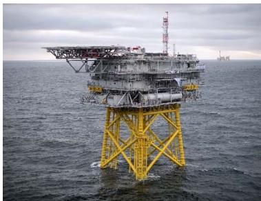
Borkum Riffgrund – installed
