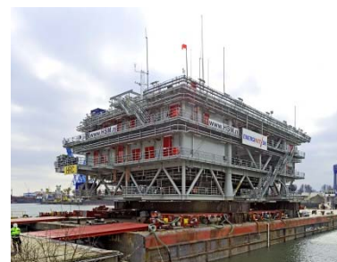
Horns Rev C - load-out
