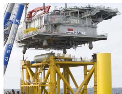
Horns Rev B - installation of topside
