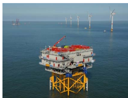
Thornton Bank - installed
